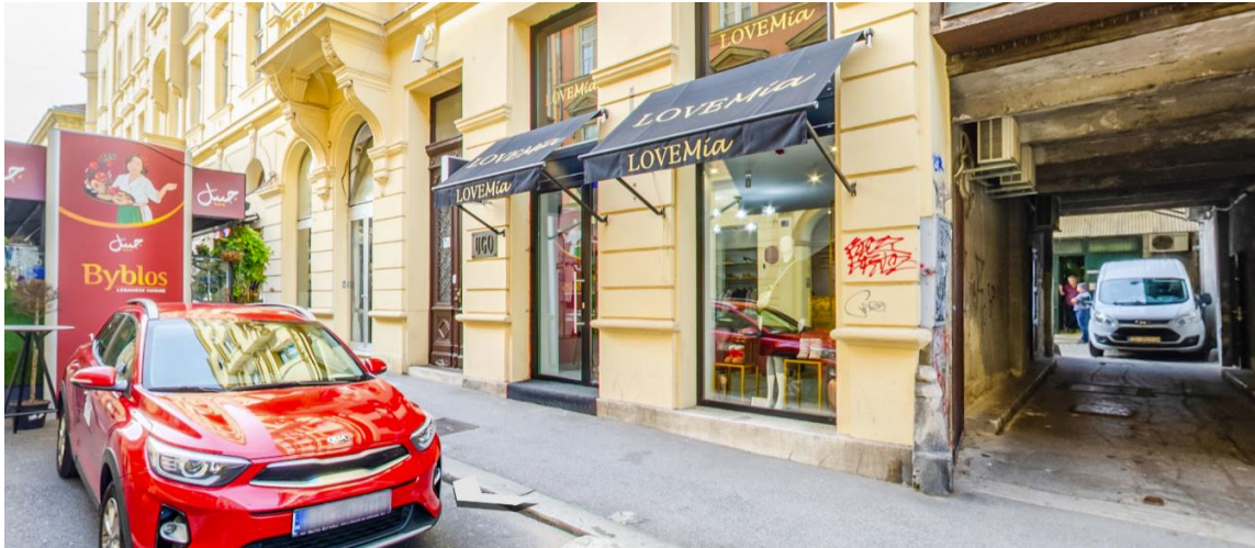
Figure 2. A repaired street-facing facade in Zagreb's Lower Town stands beside an open passage into the block interior, where the deeper courtyard condition remains largely hidden from public view. Zagreb, Croatia. Imagery © Google Maps, accessed July 4, 2026
